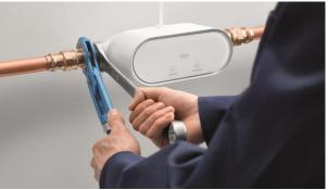
The GROHE Sense water sensor measures the room temperature and humidity, detects water retention and sends alerts when readings are abnormally high or low. GROHE Sense Guard goes one step further: Installed directly to the main water line, it can automatically turn off the water supply if, for example, a leak has been detected.
