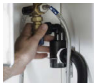
Fix safety group with holder to the cabinet and connect to the filter head outlet.
