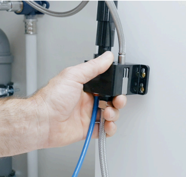
05 CONNECT SUPPLY HOSES TO THE DISTRIBUTION BOX AND ATTACH IT TO THE WALL
