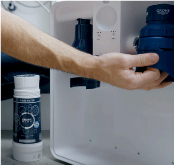
07 FINAL ONBOARDING OF THE DEVICE (FILTER, WATER + POWER SUPPLY, CO 2 )
