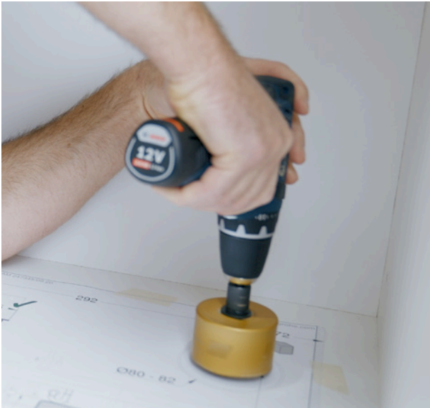
03 SAW THE OPENING FOR THE VENTILATION OF THE DEVICE
