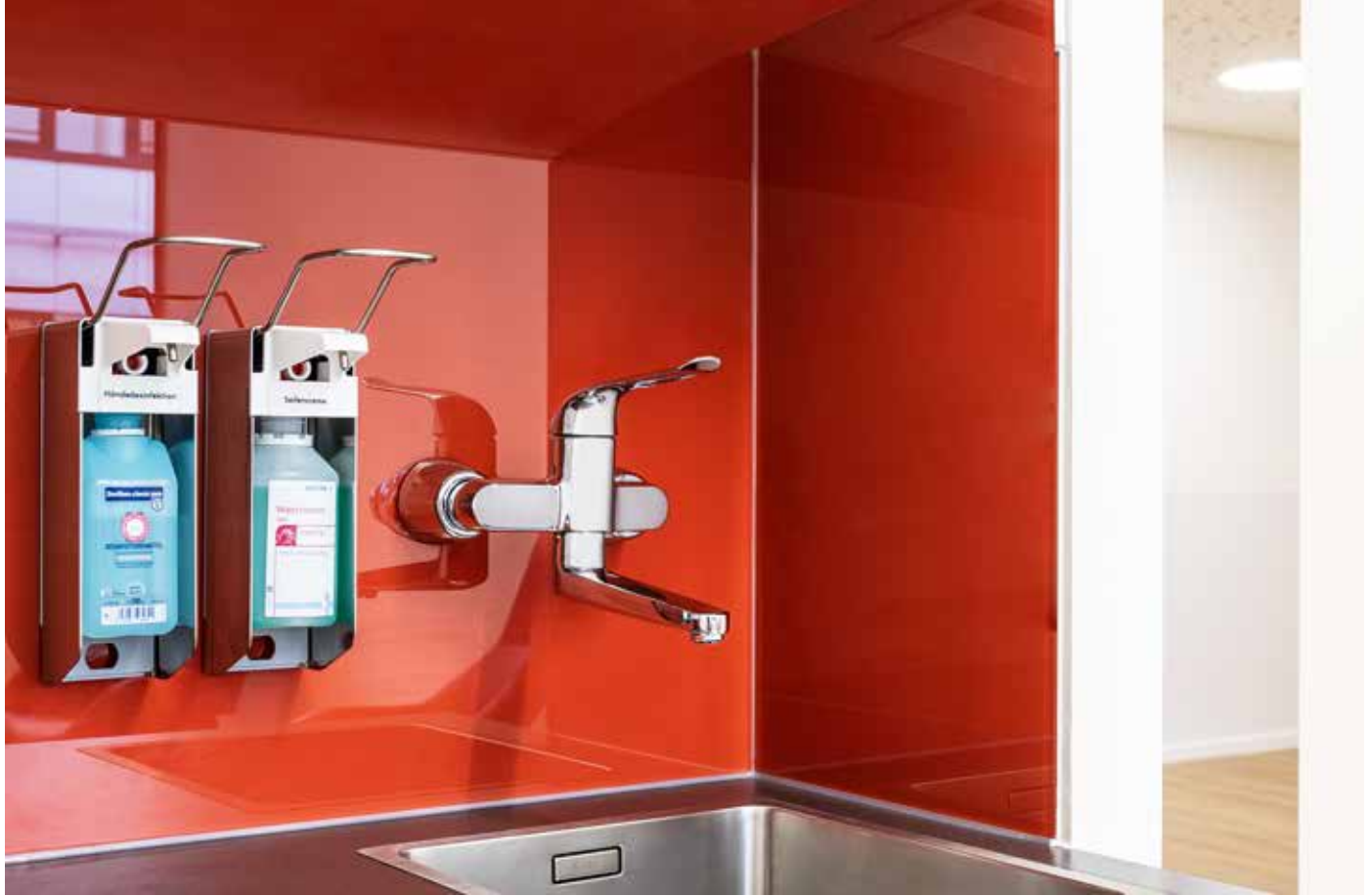
In patient treatment rooms, GROHE Euroeco special safety mixers have been specified; all the functions can be effortlessly controlled by the clinician's elbow – minimizing the risk of germ transmission and maximizing hygiene.
