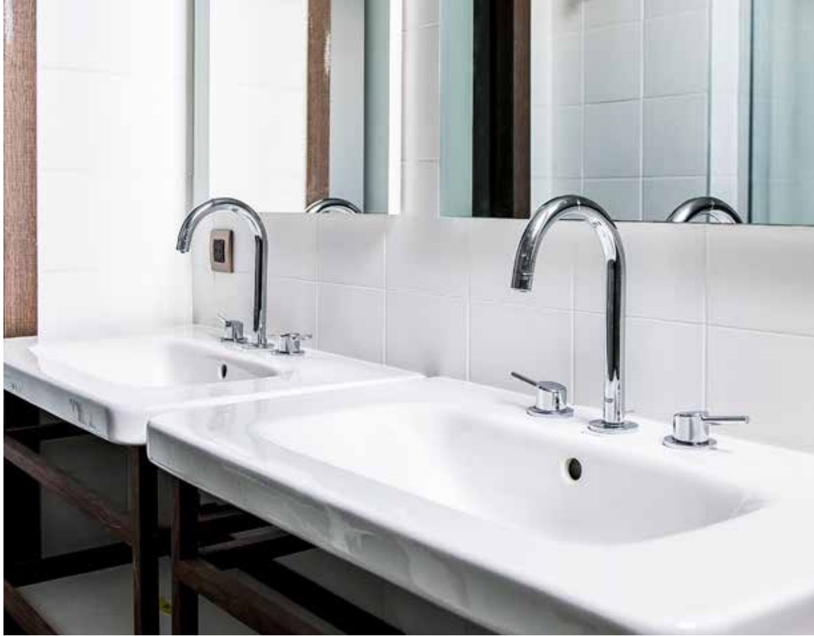
The classic, modern bathrooms at Relais de Chambord have been equipped with GROHE Concetto three-hole basin mixers in the elegant and timeless chrome finish.
