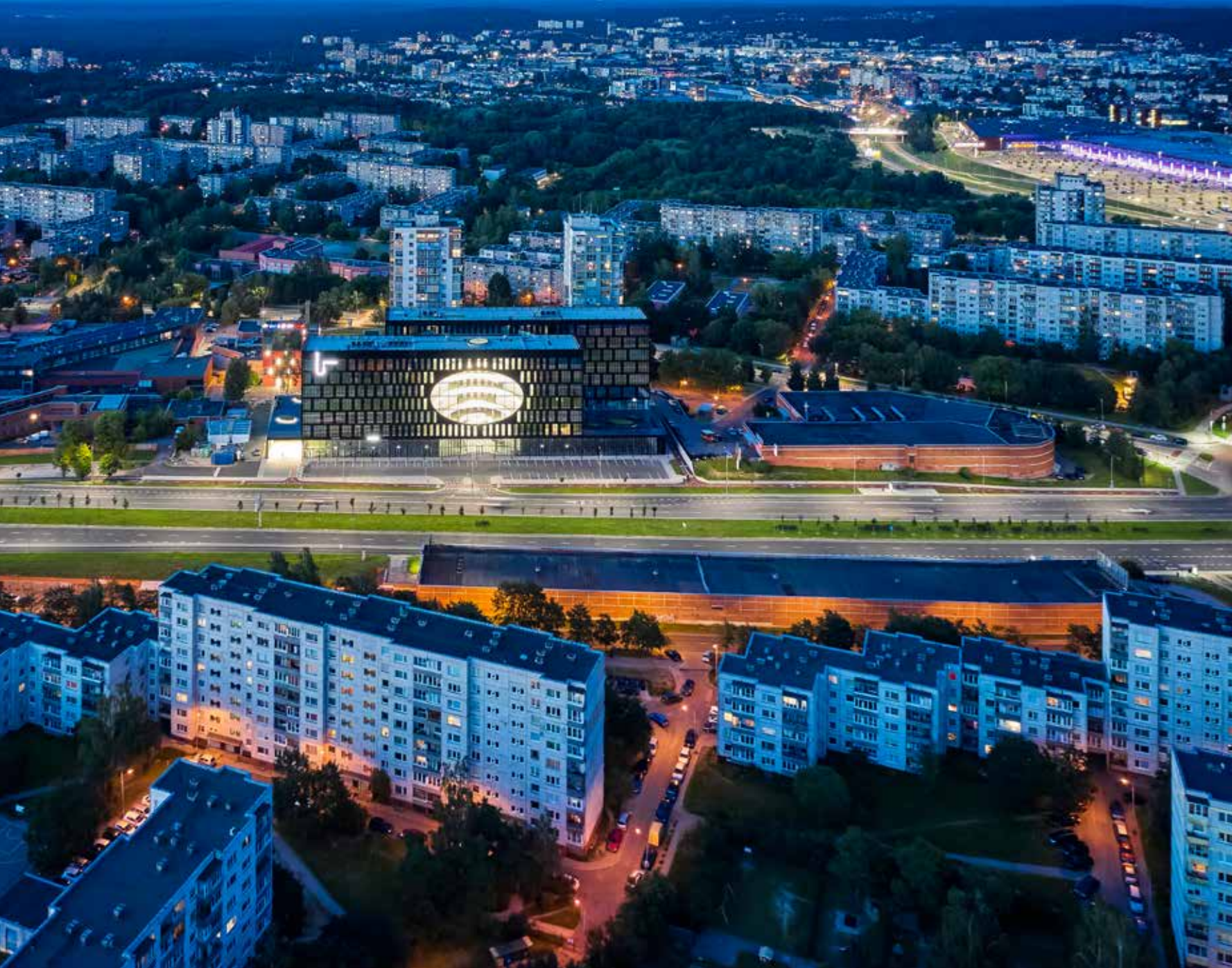
The front façade is dominated by a huge elliptical aperture. U219's defining architectural feature, it illuminates the central atrium and offers passers-by an intriguing perspective on the inner workings of the business center.
