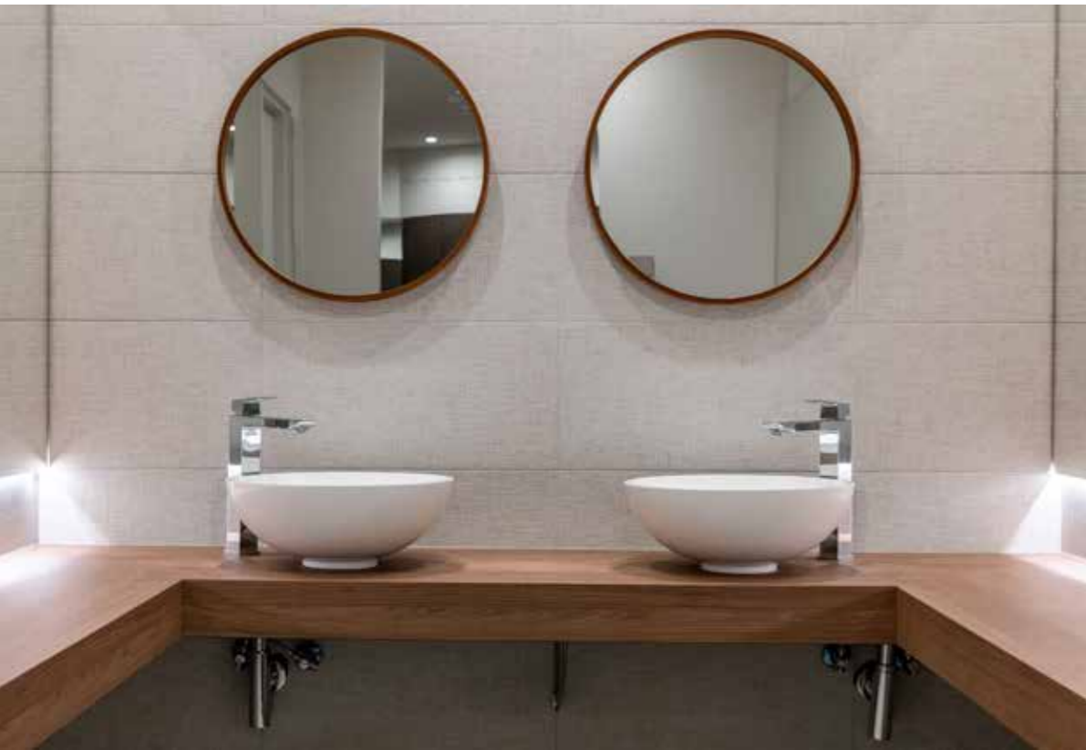
Ceramic basins in the washrooms are served by resource-efficient GROHE Eurocube single-lever mixers. Incorporating GROHE EcoJoy technology they offer an extremely precise water flow in conjunction with consumption reductions of up to 50%.
