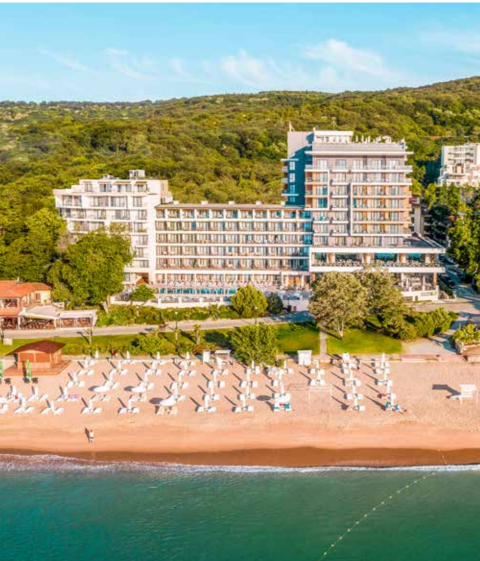
The Griffid Hotel Vistamar occupies a prime beachside location in the Golden Sands resort. The luxurious bathrooms in the suites and guest rooms of this 325-room hotel are equipped with GROHE Essence mixers and Skate Cosmopolitan fittings.
