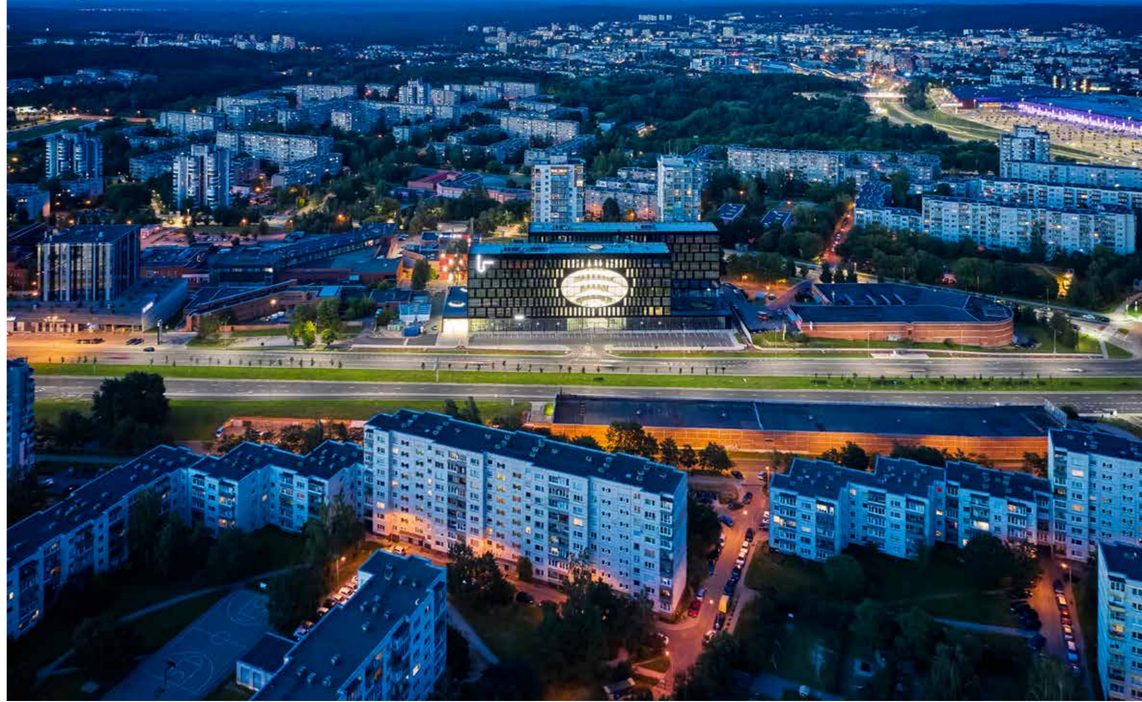
The front façade is dominated by a huge elliptical aperture. U219's defining architectural feature, it illuminates the central atrium and offers passers-by an intriguing perspective on the inner workings of the business center.
