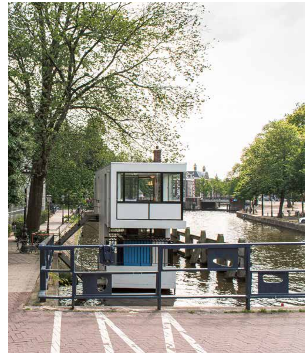
The individual architecture of each bridge house provides Amsterdam's Sweets Hotel with a unique character; for Space&Matter it also created the greatest challenge. Designing comfortable, functional living spaces required both ingenuity and flexibility.
